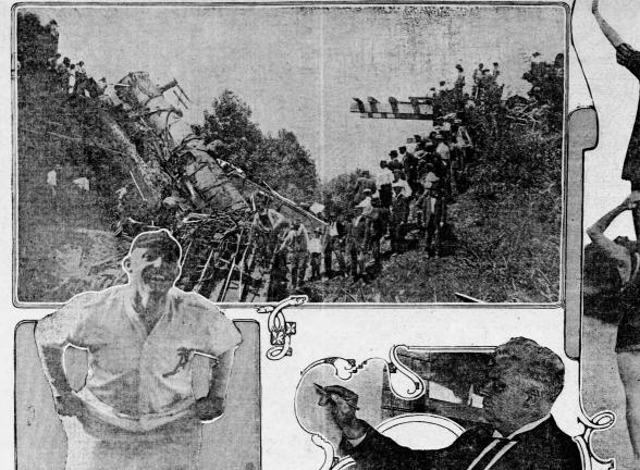
THE photograph at the top of the page shows the wreck which occurred recently near Marietta as the result of a washout. The tracks popped in two as though the steel rails had been brittle weed, and the engine was given a bad fall and was left standing almost upright. Shortly after this weed, a rearred collision happened at Scottdaie.
