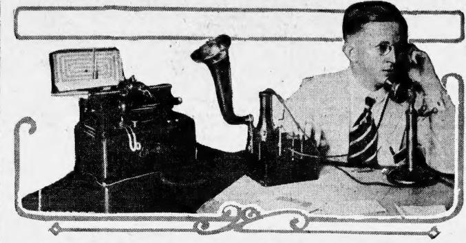
THE TELESCRIBE IN ACTION. Arthur H. Massey is shown using the machine in the office of the Baylis Office Equipment company, on South Broad street. Mr. Massey is seated at the ordinary telephone. He has taken the receiver off and clamped it on the Telescribe, using another receiver attached to the Telescribe to hear through. At his extreme right is the dictating machine equipped with a record which is catching every word uttered by Mr. Massey and the party on the other end.
