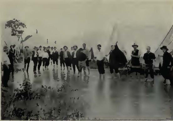
MAIN STREET DURING FLOOD
